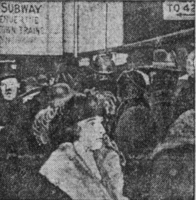
A crowded, unheated, and unlighted subway station where going to and from their jobs, the wage earners of New York may yet be compelled to pay a seven-cent fare if the traction magnates succeed in their present campaign. Photos show scenes at subway stations with subway "patrons" getting ready for the daily scramble.
