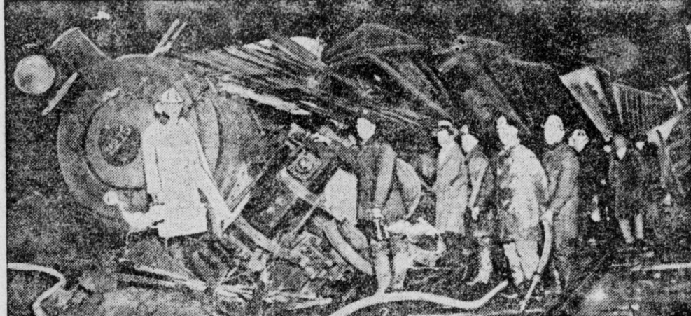
This photograph shows the wreck of a locomotive and part of the freight train it was hauling after the train had buckled across the tracks near Washington, D. C. The driver of the locomotive was killed in the wreck. The blame for such wrecks is usually placed on the engineer, who is not alive to defend himself, even though the railroad is to blame.
