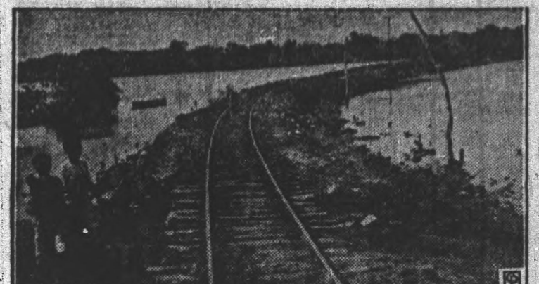
A heavy marine guard is being maintained at this bridge at Corinto, which, if destroyed by a bomb, would cut the only rail connection between the marine base at Corinto and the interior. Corinto workers are aiding the Sandino forces in their struggle for Nicaraguan independence.
