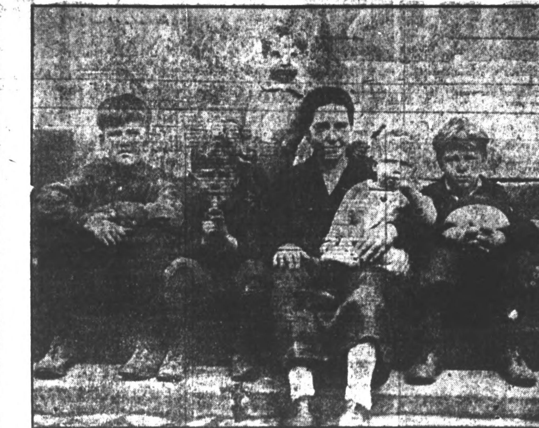
The Equitable Gas Co. of Pittsburgh on Monday morning put a crew of men with torches to repair a gas tank into which they let some gas. The men supposed the tank empty. The resulting explosion killed about fifty men, workers on the tank and in the pottery works next door, and wounded an unknown number, amounting to several hundred, of the working class residents and passers-by in the district. Photo shows babies' bandaged heads—cut by steel projectiles from the explosion. The workers' homes in the neighborhood were destroyed by the blast.
