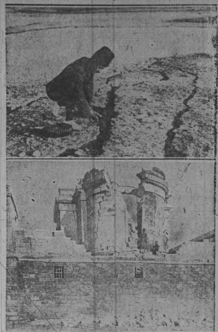
First pictures of some of the results of earthquake in Palestine, originating in the Dead Sea region, causing the loss of more than 400 lives: Top, one of the deep fissures at the Dead Sea caused by the heavy tremors. Below, ruins of the newly constructed winter palace at Jericho. In this building, three Indian tourists were killed and buried.
