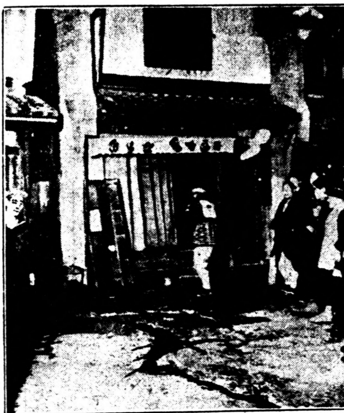
Photograph just received of effects of the recent Japanese earthquake—a gaping crack in an Osaka street.
