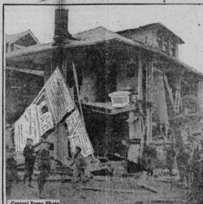
When an explosion of natural gas wrecked a residence in Canton, O., the owner, who was in the bathroom, was blown thru the side of the house out into the yard. His wife and their young child were in a room on the second floor of the house when the floor fell, dropping them to the first floor. None was seriously injured. Workers in the street had turned off the gas line to repair the street and the explosion occurred when the gas was turned on again. This danger is a constant menace to workers' homes, almost exclusively utilizing gas. Electric improvements would obviate these dangers.
