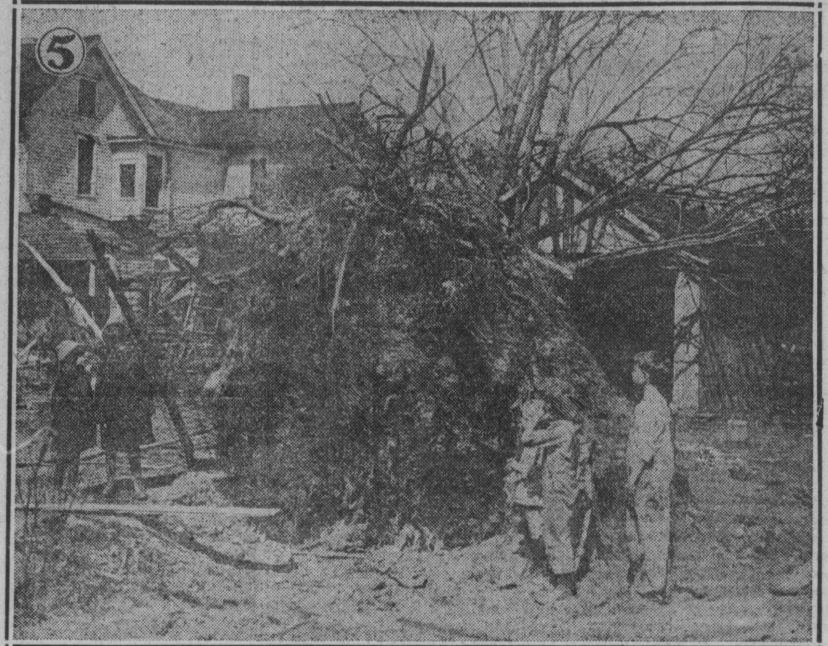
The powerful wind, that uprooted giant trees, played havoc with the shacks that served many of the workers as homes. The better constructed houses stood against the storm.
