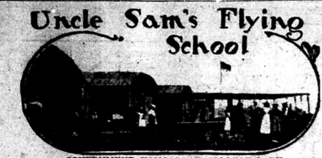
GOVERNMENT HANGAR AT COLLEGE PARK.
