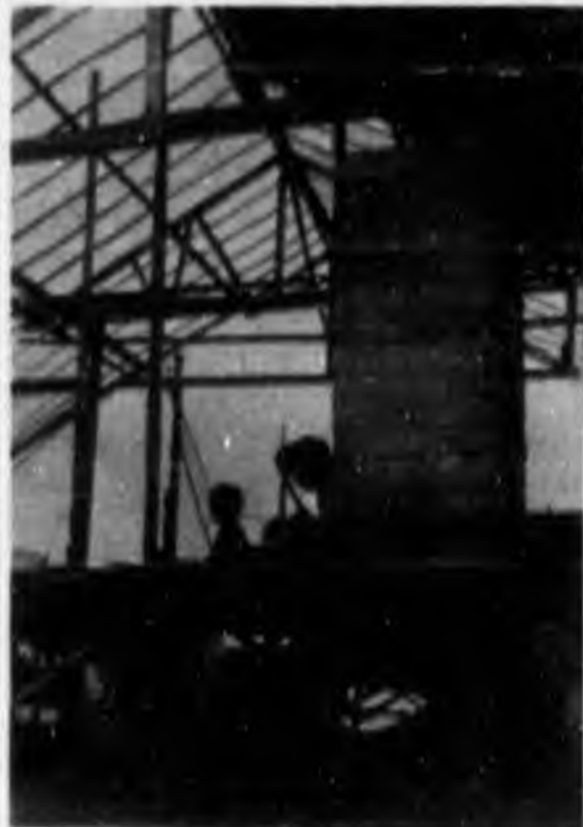
A house stripped bare in hamletted area
