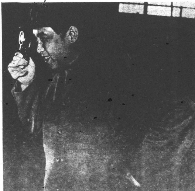
Premier Kim Il Sung inspecting iron works
