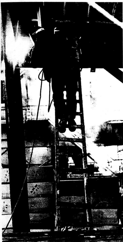
The ladder is not secured and has a rung missing. One false step and this welder could fall on blowtorch.
