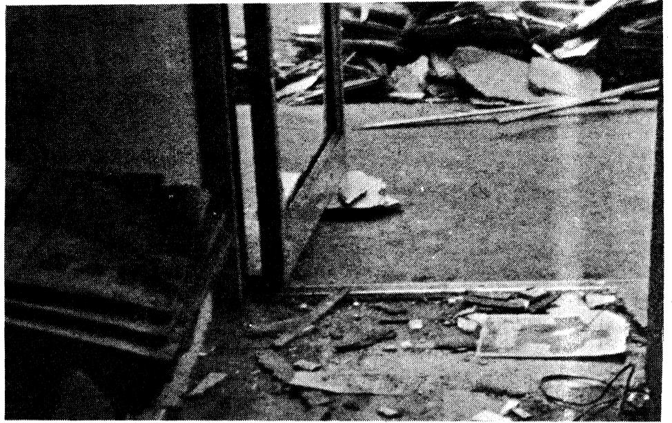
Part of damage done to Socialist Workers Party campaign headquarters by March 12 bombing.
