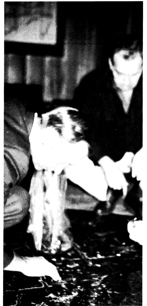
FIRE-DAMAGED FLOOR. L.A. socialists were target of New Year's Eve terrorist attack.
