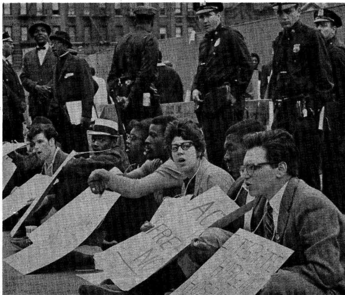
JOB-RIGHTS SIT-DOWN. To emphasize demand for end of discrimination in building-trades hiring, a group of pickets sit down at approach to construction site of new wing of Harlem Hospital in New York. City administration, which has recently grown sensitive to civil-rights demands, ordered job shut down pending negotiation of issue.
