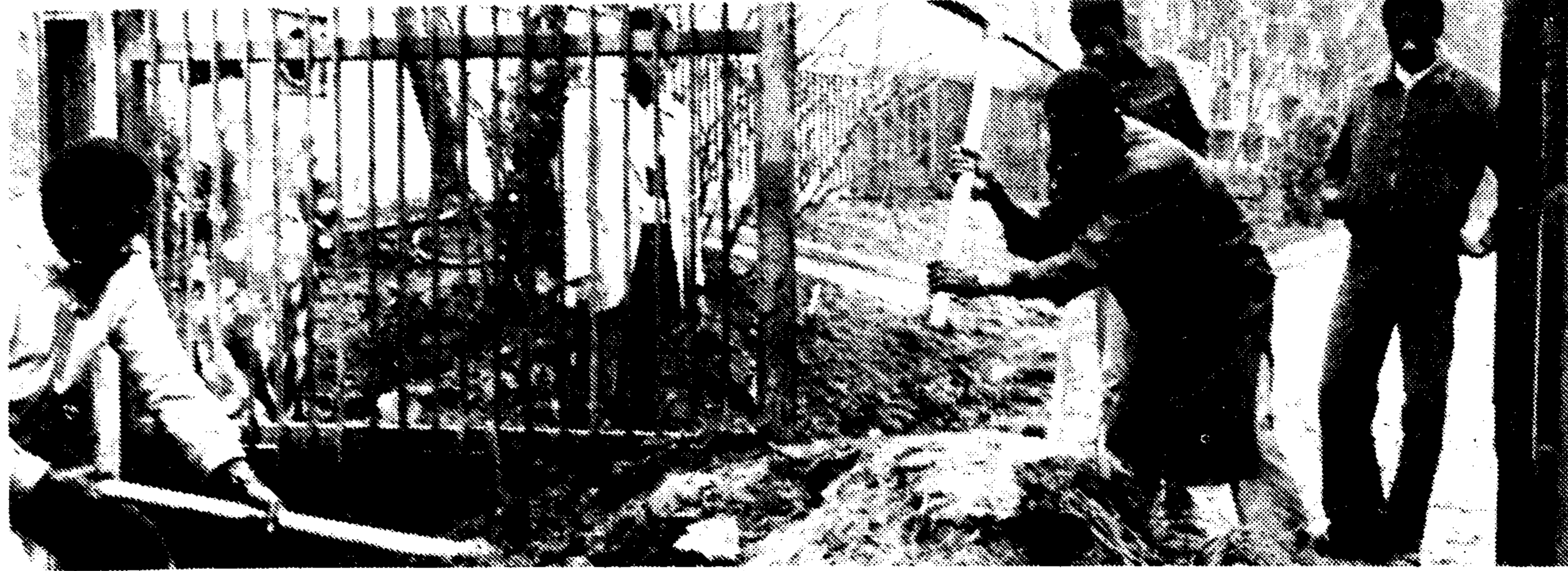
Mali workers repair damage done by Stalinist raid
