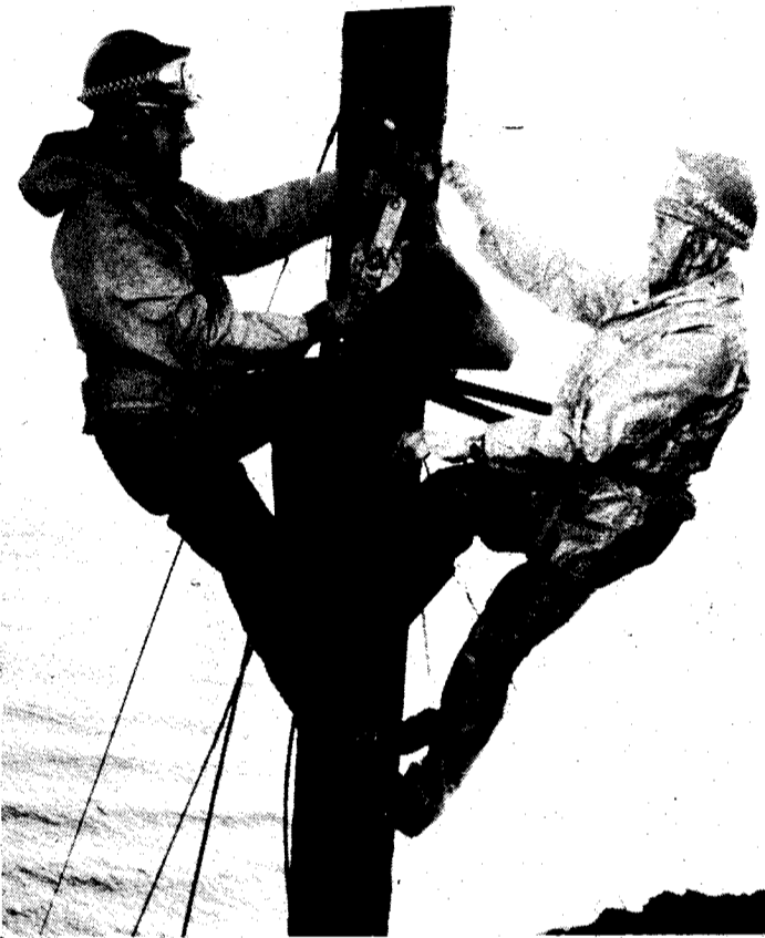
Telecoms engineers: don't leave them without support
