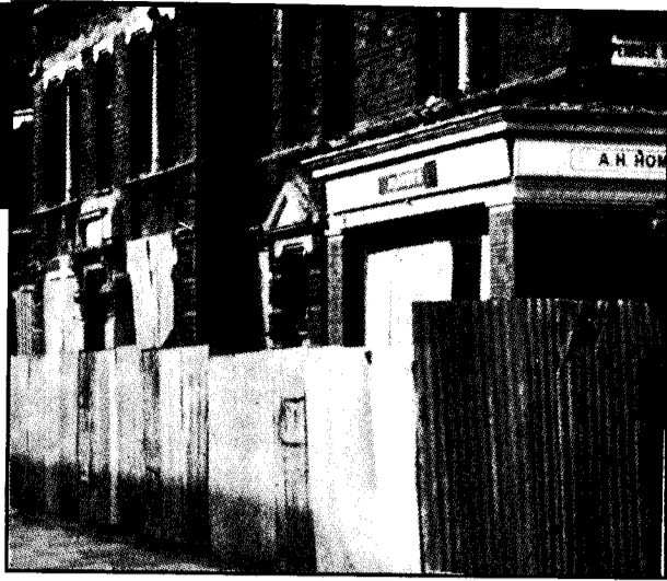
Corrugated iron screens urban decay in Southwark
