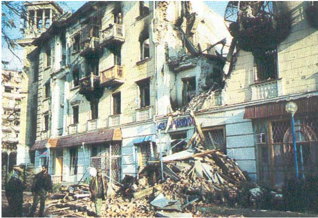
Bombed house in Grozny, 1999
