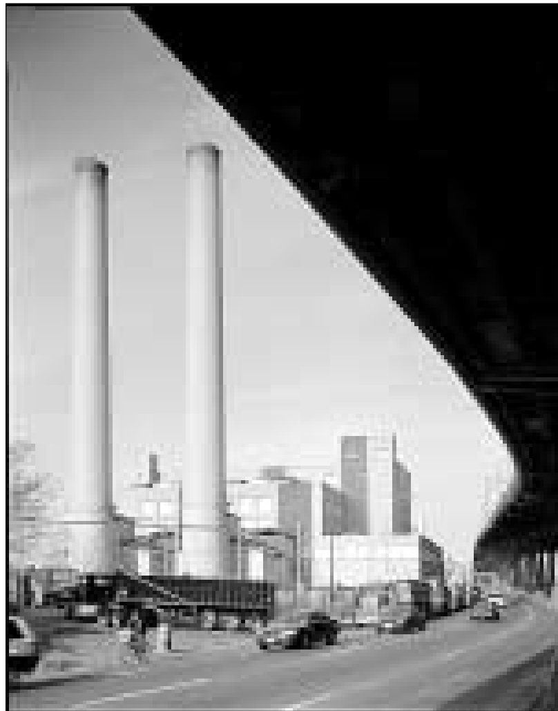
New York incinerator: Hazard and charges
