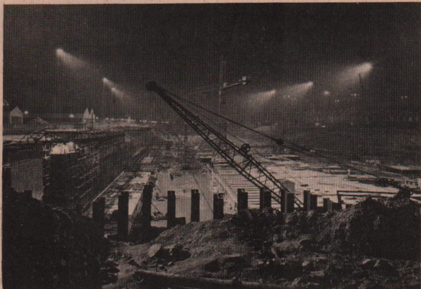
Building a new dock by night
