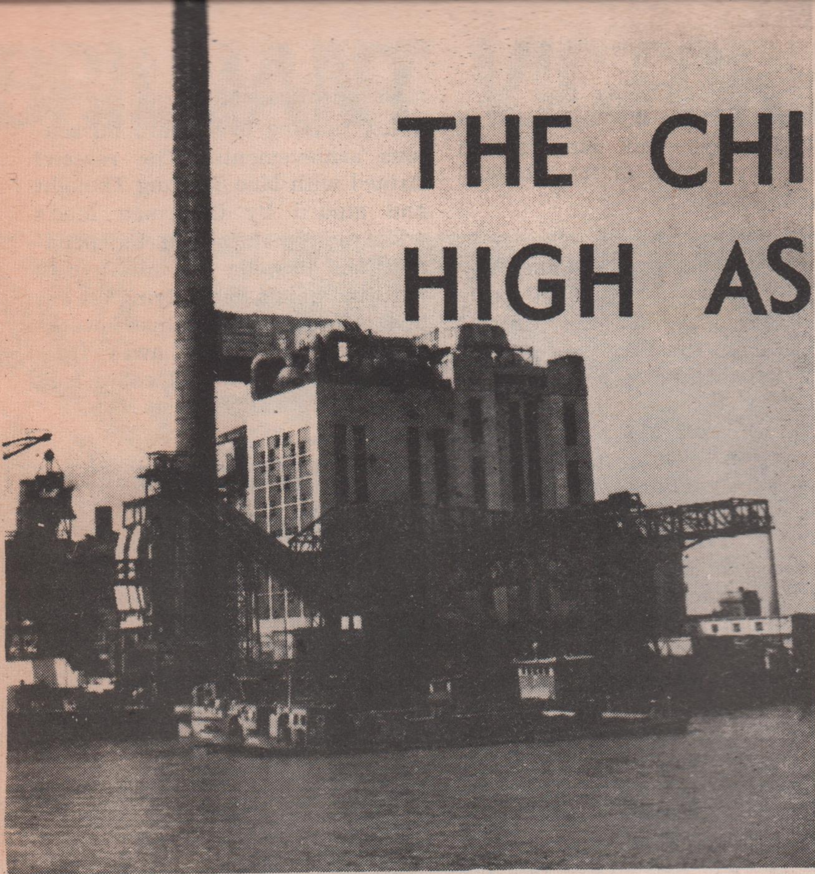
The Yangshupu Power Plant.
