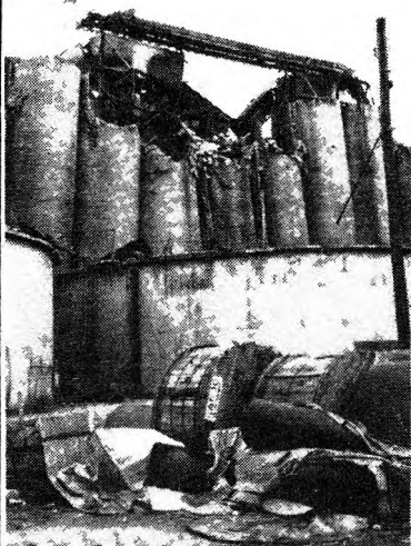
Aftermath of deadly explosion at Continental Grain Company Since then three other major explosions have taken place
